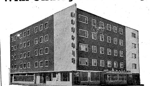
The Mayfair's clean, contemporary exterior elevation is designed so as to eliminate the necessity of exterior maintenance, and features terrazzo and masonry construction, Italian marble on the north and east walls, providing a rich contrast to the upper masonry walls, and all-metal windows, screens and storm sash. The door frames, base and window trim are also of metal.
